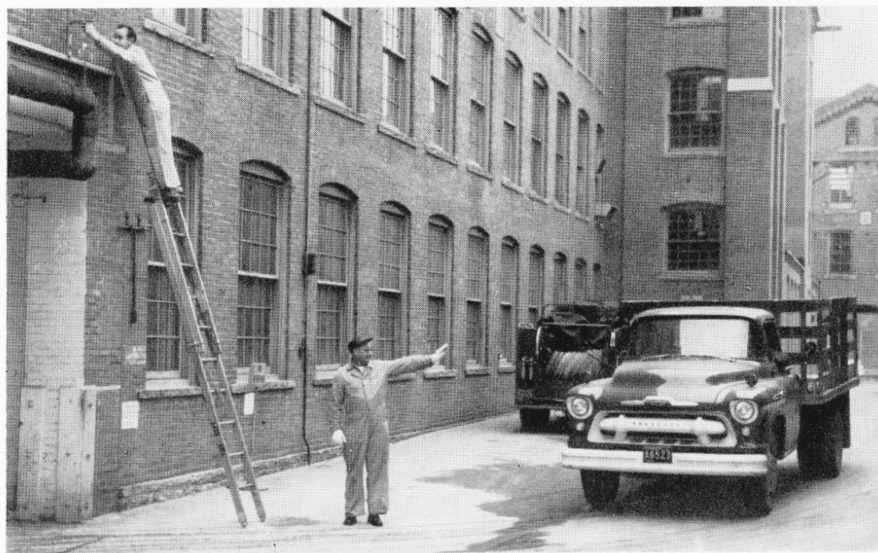
Whenever ladders are used in the vicinity of moving objects, the base should be protected as demonstrated by fire inspector John Niedmann. John directs moving traffic away from the ladder while Cliff Aspinall is on it.
